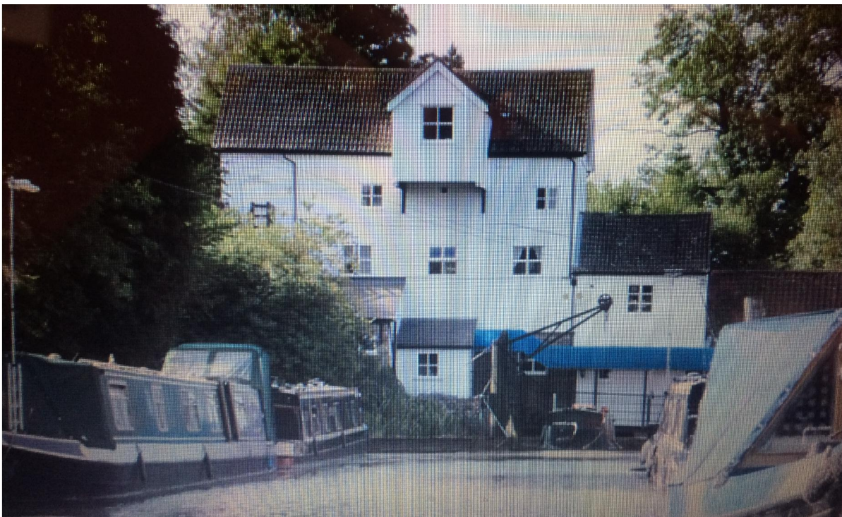
Little Hallingbury Mill viewed from the Marina.
